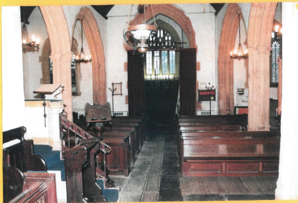
3. Nave & Tower Arch. Looking West.
